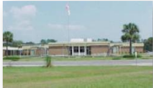
Blountstown Elementary School http://www.blountstownelementary.org/
